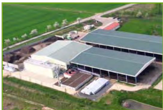
Waste fermentation plant in Weißenfels
